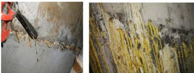
Figure 4. Roof and sidewall grouting.
