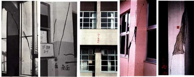
Photo. 1: Building damaged by the 1968 Tokachi-oki earthquake Photo. 2: Building damaged by the 1978 Izu-Oshima earthquake Photo. 3: Building damaged by the 1995 Hyogo-ken Nanbu earthquake Photo. 4: Building damaged by 1997 Kagoshima-ken Hokuseibu earthquake Photo. 5: Building damaged by 1997 Kagoshima-ken Hokuseibu earthquake
